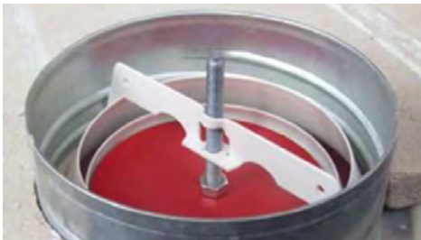
Fire rated Ceiling Air Valve installed before a fire.
