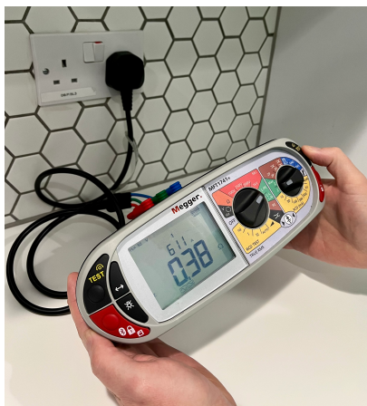
Electrical tests being carried out.
